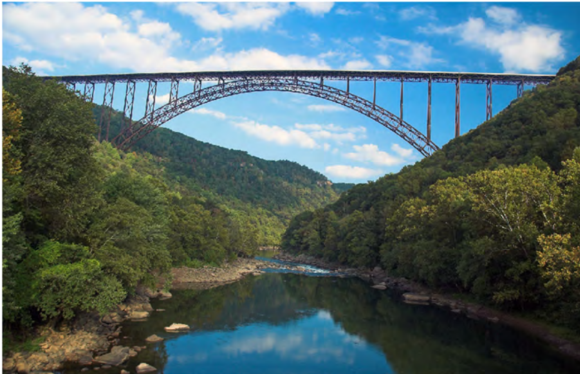
New River Gorge Bridge, National Park Service (at much lower water!)
