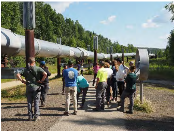
Figure 19. The Alyeska Pipeline Viewing Point. The Alaska Oil Pipeline is elevated for the most part and has cooling fins to prevent the permafrost from being impacted. It is the reason that there is essentially any infrastructure north of Fairbanks.
